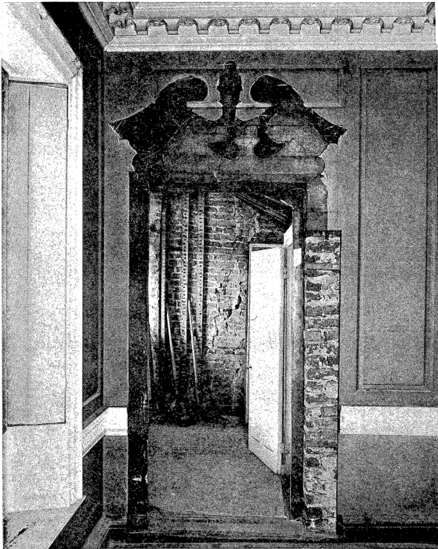
Illustration No. 13: Same door after the broken pediment had been removed.
