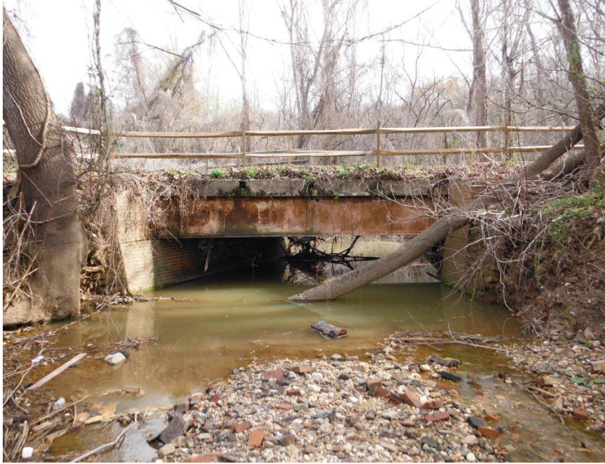
Photo 1: South (Downstream) Elevation
