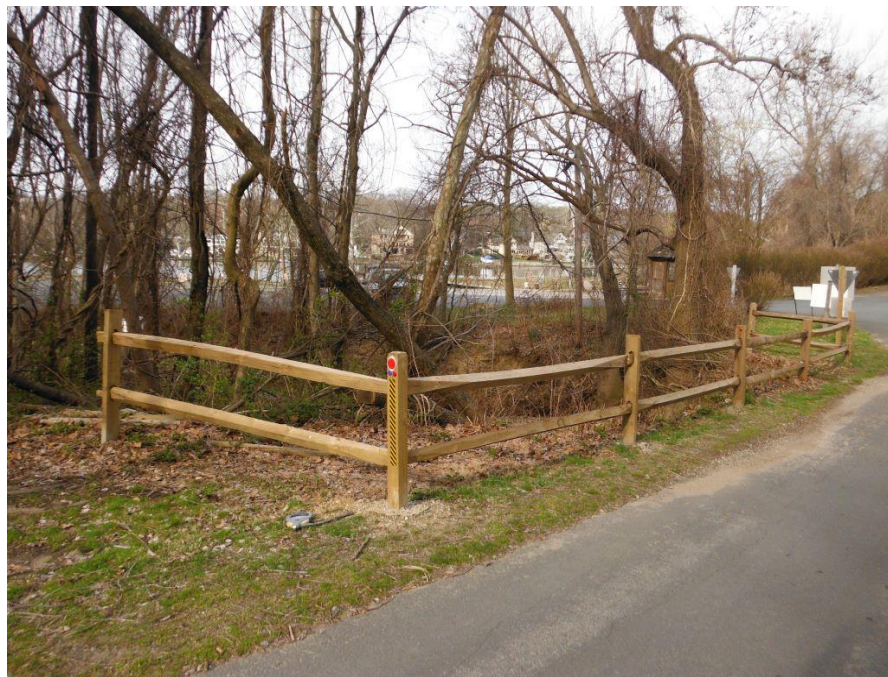
Photo 6: New timber railing on downstream side, looking from east approach
