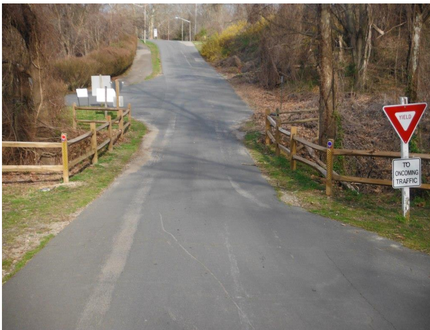
Photo 2: East Approach (Looking West)
