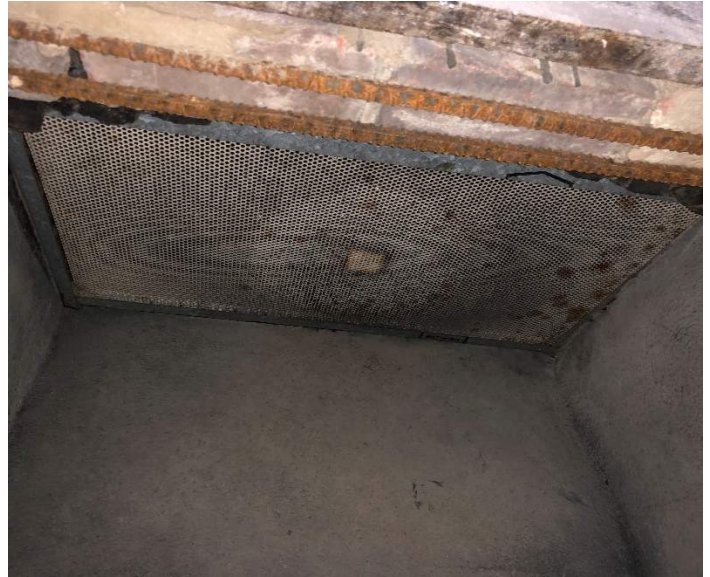
Existing Fireplace grille to be replaced provide duct transition to fully utilize perforated face for lower noise.
