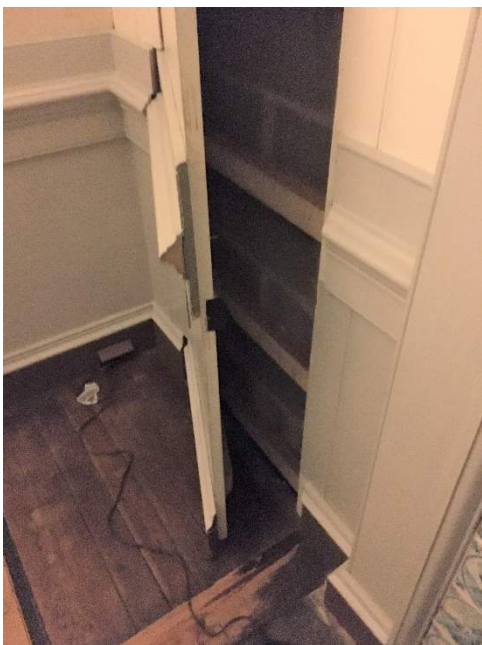
South face of CMU shaft to attic for new outside air riser, adjacent to Fireplace in Room 104
