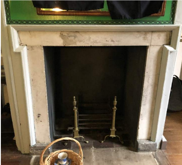
First Floor Fireplace (example). No fireplaces are functional. Flues are used to route piping and ductwork.
