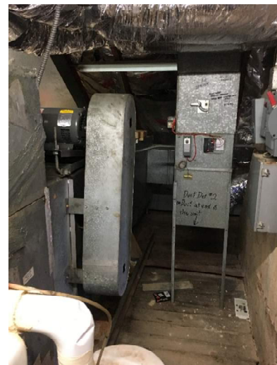
Multizone AHU to be dismantled and removed via deconstructed dormer window
