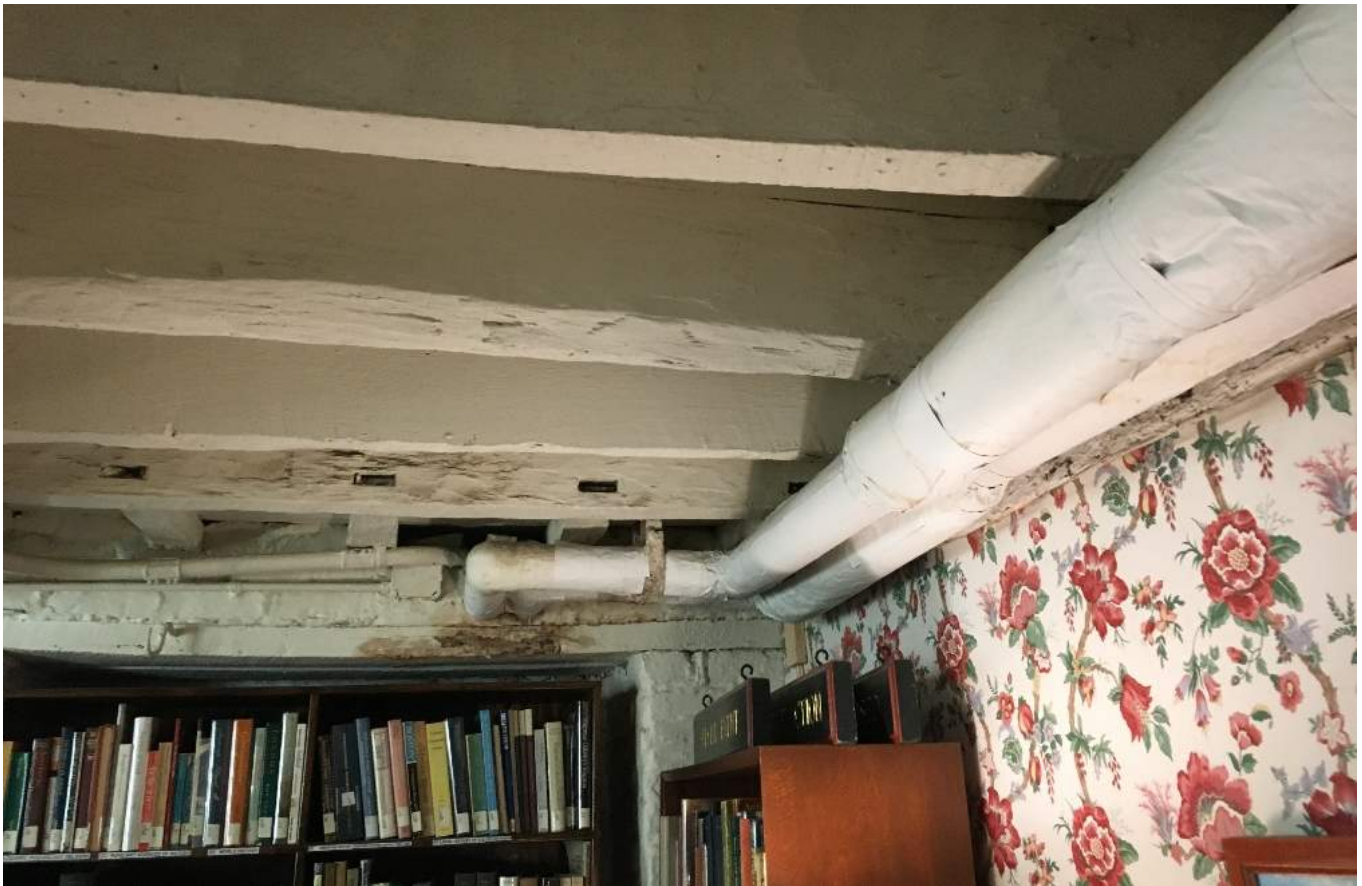
Location of existing to be removed Chilled Water piping, and location of new outside air and supply air duct penetrations to/from Basement Blower Coil Unit
