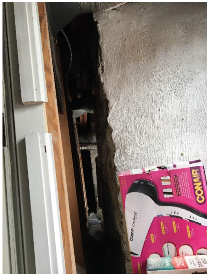
Restroom Wall Cavity, Exhaust window connections. Similar space for new refrigerant piping entrance and rise to toilet room ceiling.
