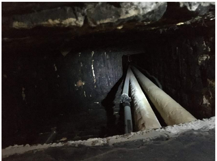
Existing chilled water supply and return piping rising to attic through fireplace flue. Piping is to be removed.
