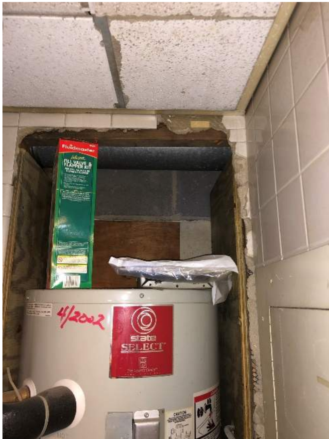
Water Heater closet, fireplace CMU shaft to attic for new outside air riser
