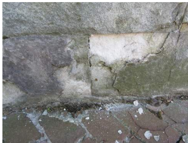
Figure 46: Flaking face of stonework.
