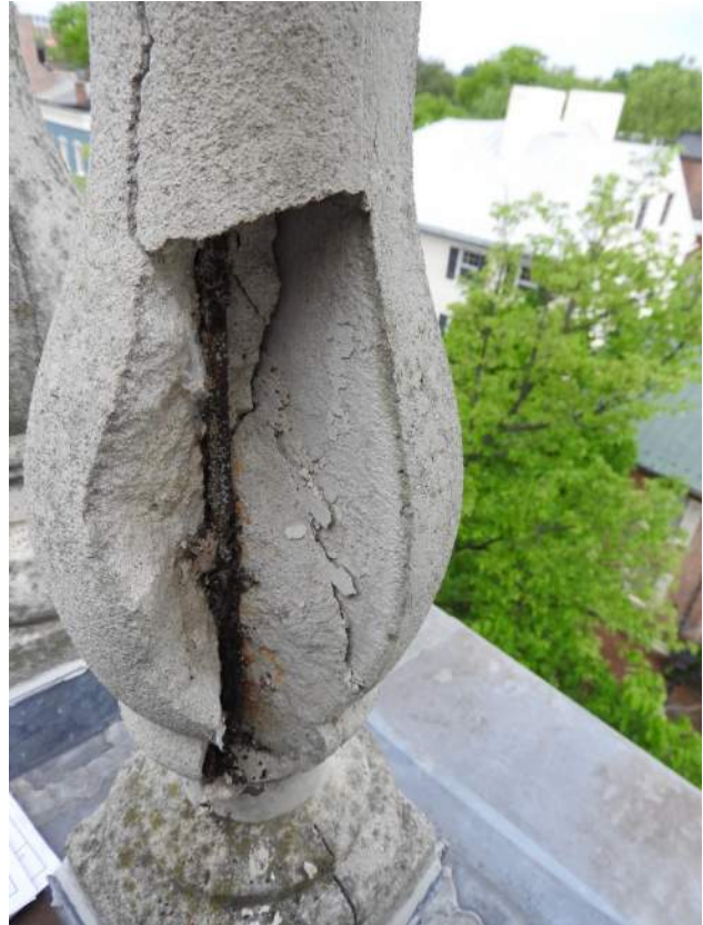
Figure 17: Spall at baluster exposing interior metal rod.
