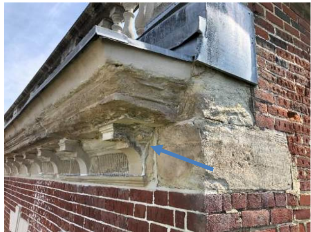
Figure 22: Remnants of historic limewash on face of bracket.
