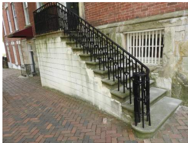
Figure 50: North stair construction with stucco coating.
