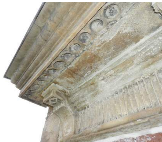
Figure 9: Cornice and frieze detailing, viewed from below.
