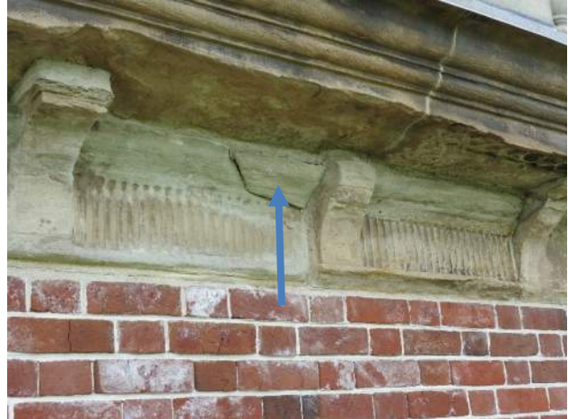
Figure 27: Loose stone at north frieze detail noted prior to removal.
