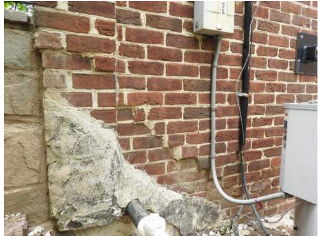
Figure 42: Separation in existing brick construction.
