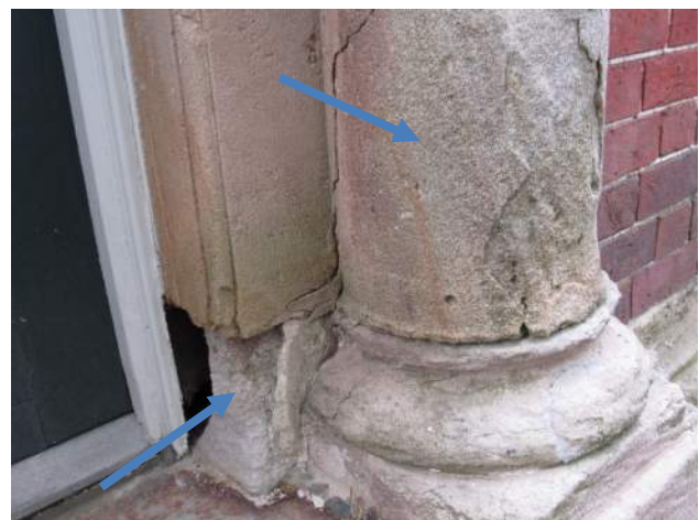
Figure 54: Stone deterioration at north stone surround.
