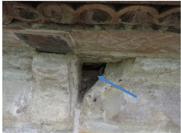
Figure 28: Area of removed stone at north elevation frieze detail.
