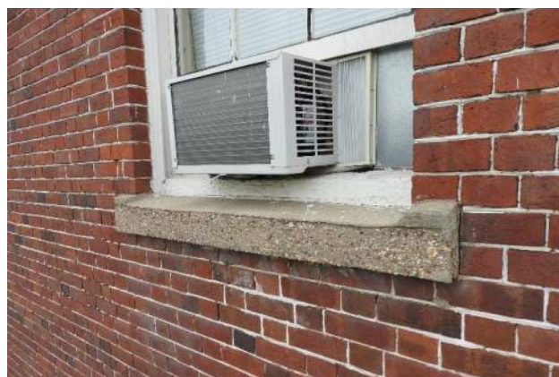
Figure 30: Typical replacement concrete sill with cementitious parging at topside.
