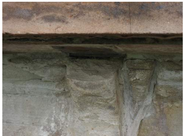
Figure 23: Loss of bracket, signs of exfoliation, and past patching efforts at bracket location.
