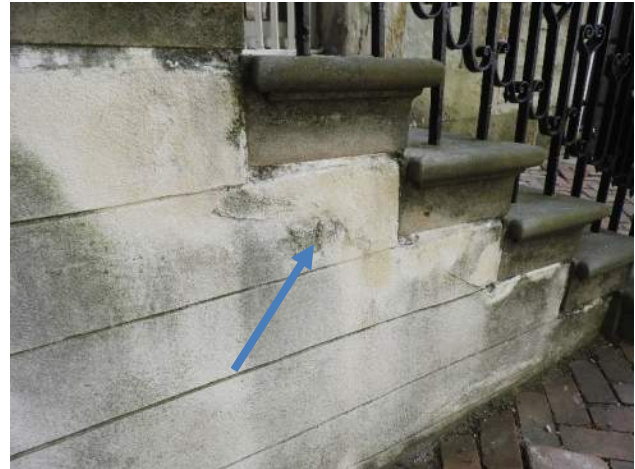
Figure 52: Cracking and loss of finish coat in stucco.
