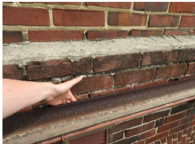
Figure 57: Observed gap at roof terrace gutter system.
