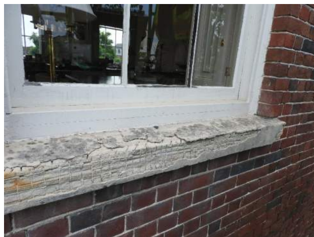
Figure 34: Surface staining and failing patching at stone lintel.
