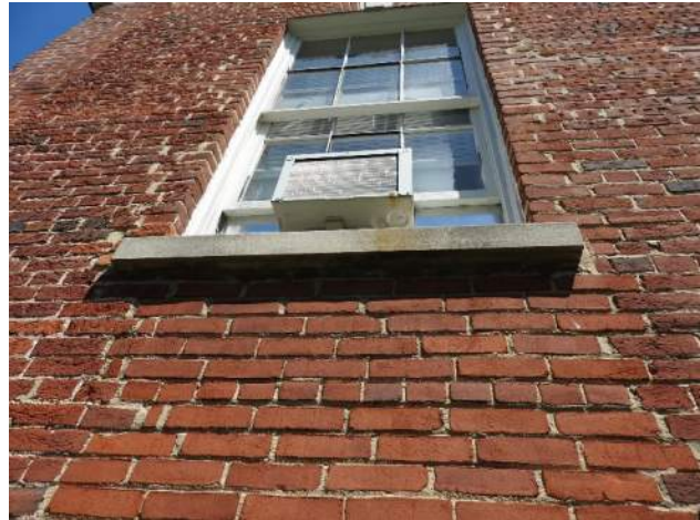
Figure 38: Typical modern cast concrete sill on south and east elevations.
