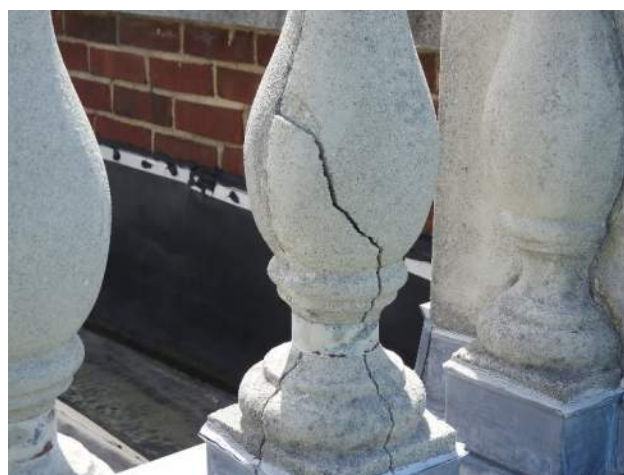
Figure 16: Typical cracking in baluster.
