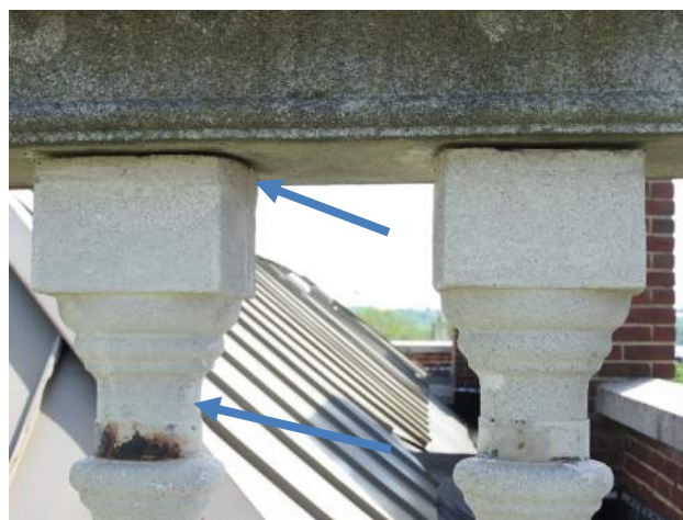
Figure 12: Top of baluster grout pad connection to concrete railing, with crimps at balusters.
