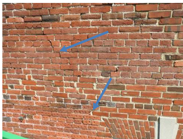
Figure 40: Existing cracking above window opening at south elevation.
