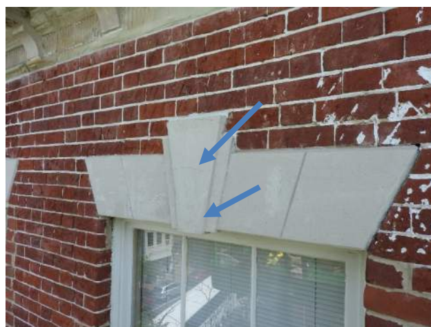
Figure 33: Cracking at face of patched stone lintel.
