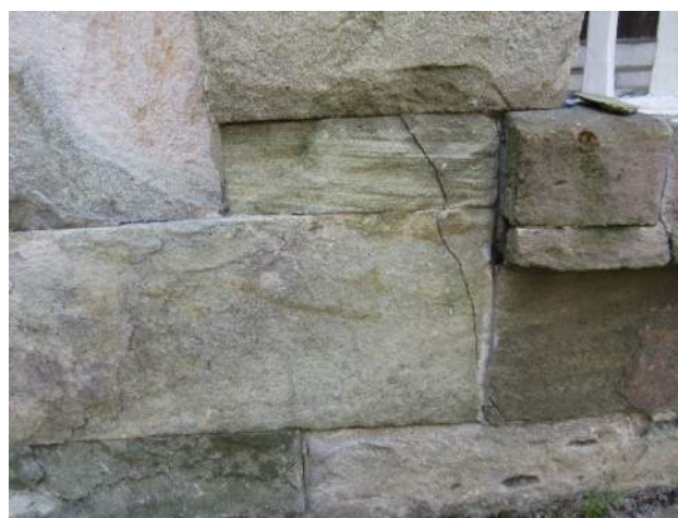
Figure 48: Cracking in stonework.
