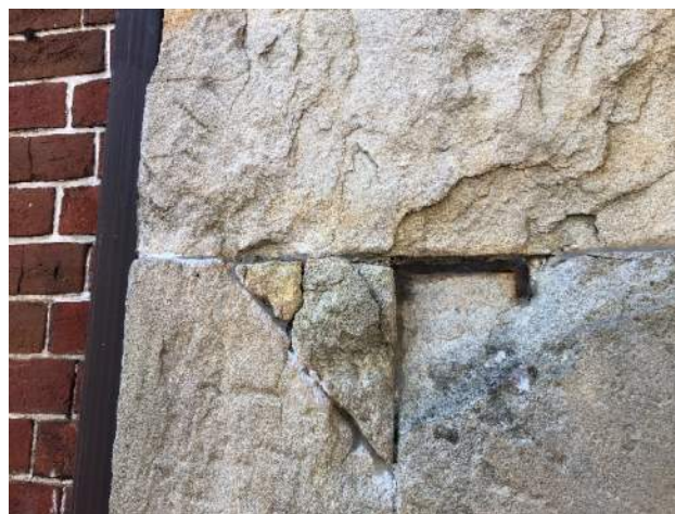
Figure 47: Spall at embedded iron tie.
