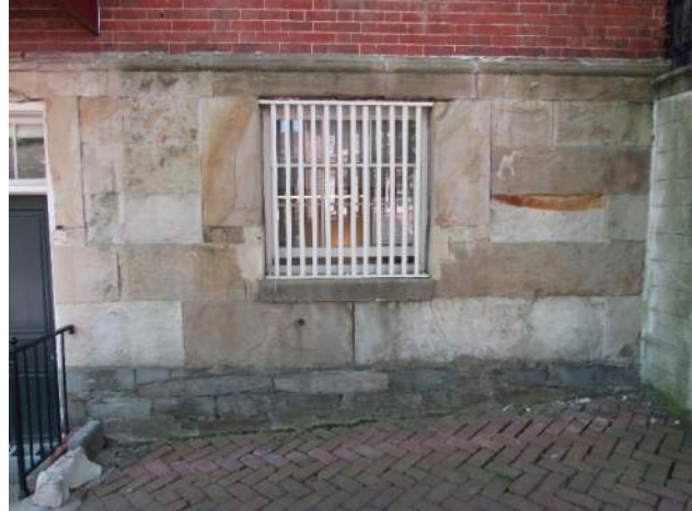
Figure 43: Typical sandstone band transitioning to bluestone on north elevation.
