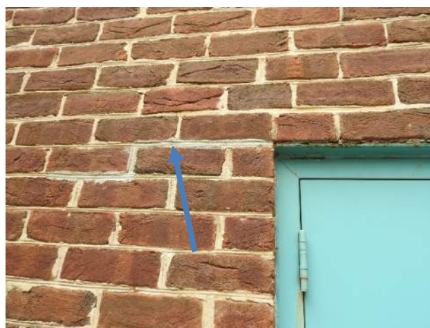
Figure 37: Recent repointing at steel lintel bearing, indicating rust jacking.
