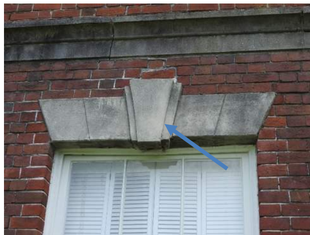
Figure 35: Slipped keystone in stone lintel on north elevation.
