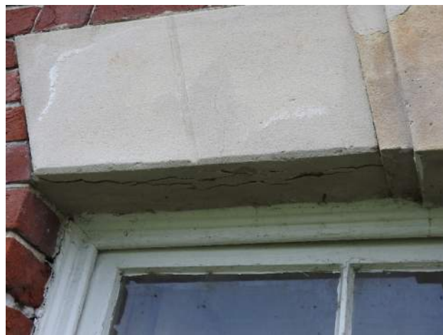
Figure 32: Cracking at underside of patched stone lintel.
