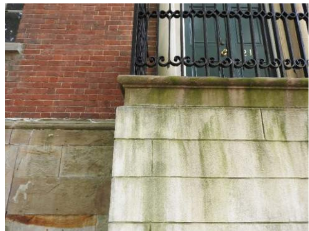
Figure 53: Typical surface staining at stair.
