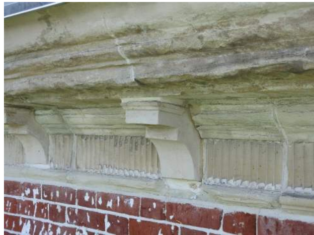
Figure 25: Replaced bracket detail at west elevation.
