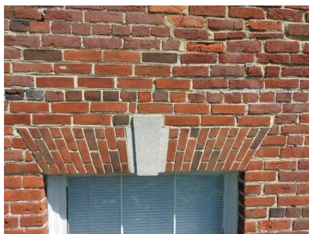
Figure 36: Typical modern lintel configuration at south and east elevations.
