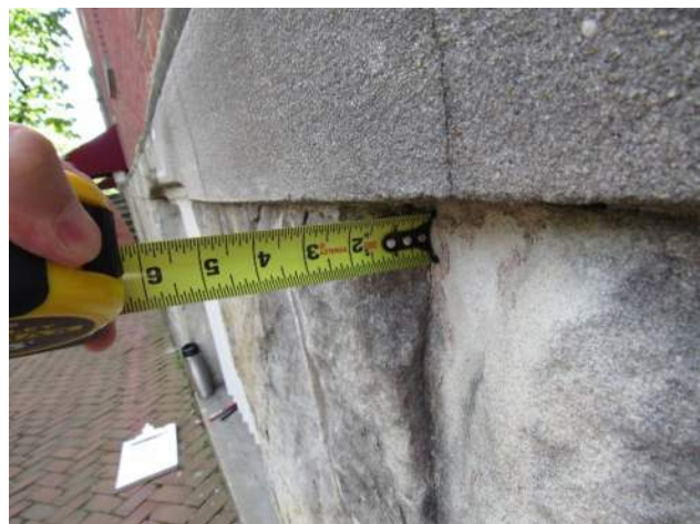
Figure 45: Existing spall at north face.
