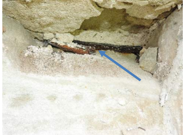
Figure 21: Remnants of iron tie at removed stone.
