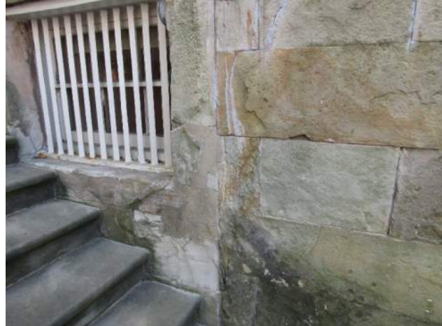
Figure 49: Surface staining from biological growth and previously caulked joints.
