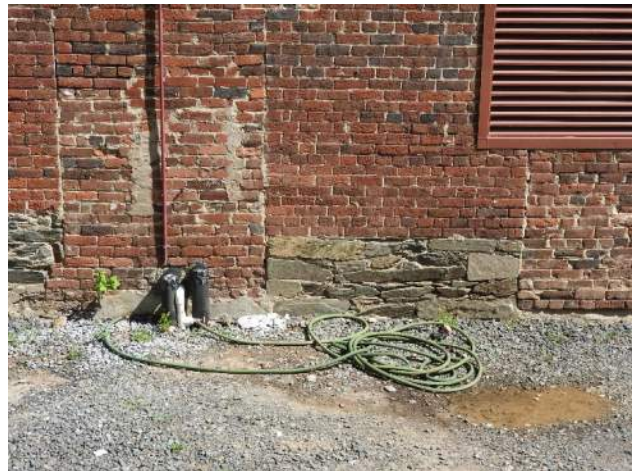
Figure 44: Granite at base of brick on south elevation.
