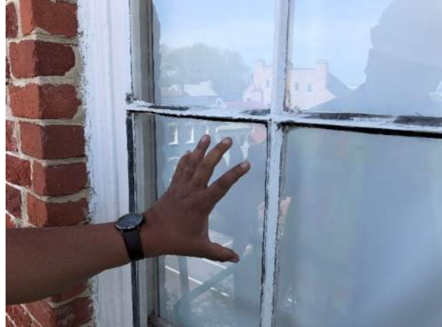
Figure 55: Loose windowpane, muntins with mold growth.
