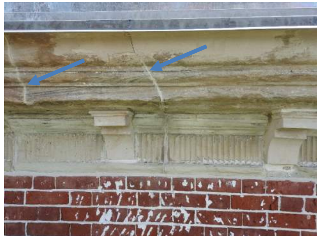
Figure 26: Stone with open cracks and cracks with some evidence of past repointing.
