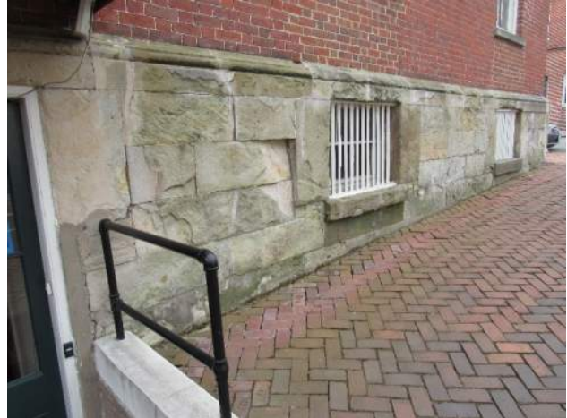
Figure 5: Sandstone band at base of wall on north elevation.
