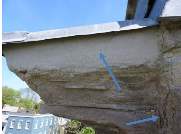
Figure 24: Stone flaking and past patching efforts at southwest cornice detail.
