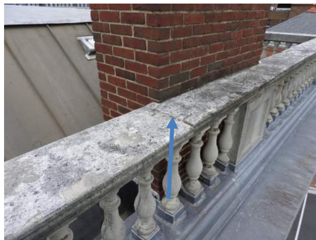
Figure 11: Top side of balustrade assembly, with cramps visible.
