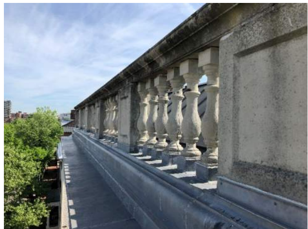
Figure 7: Cast concrete balustrade on west elevation.
