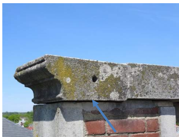
Figure 13: Rotation of concrete coping away from west elevation.
