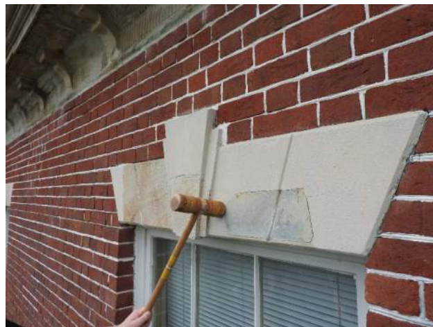
Figure 29: Typical stone lintel with patching.
