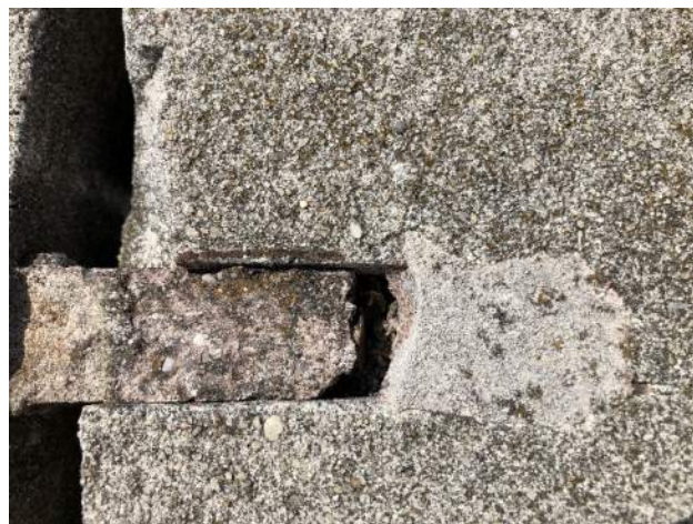
Figure 14: Failed crimp and separation between rail stones at west elevation.
