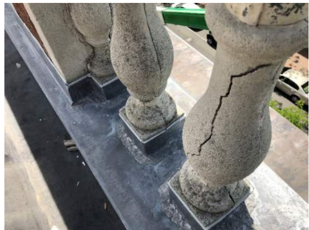
Figure 18: Flashing detail at base of balustrade assembly and at base of individual balusters.
