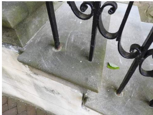
Figure 56: Typical railing embedment at stone treads.
