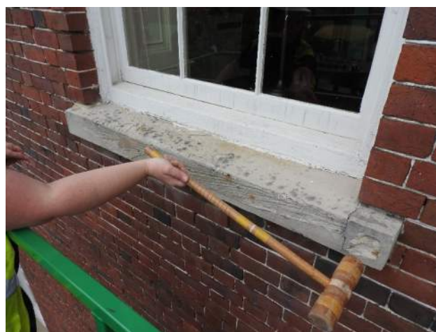
Figure 31: Sounding stone and patches at existing sill. Cracking in sill at edge of patching material.
