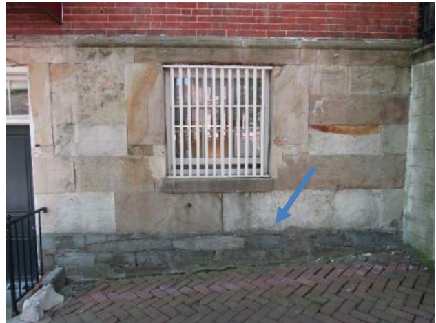
Figure 6: Sandstone band transitioning to bluestone.
