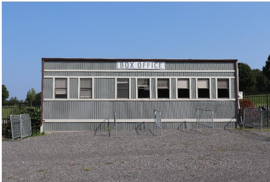
Box Office Exterior
