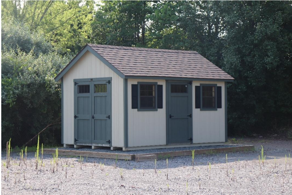
Event Storage Shed
