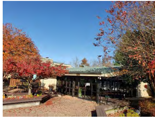
E-6: Roof 1 – East
