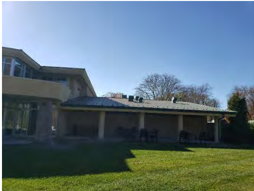
E-13: Roof 5 – Overall
