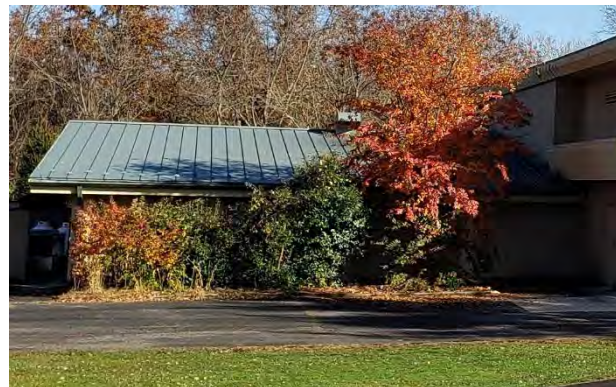
E-12: Roof 4 – West
