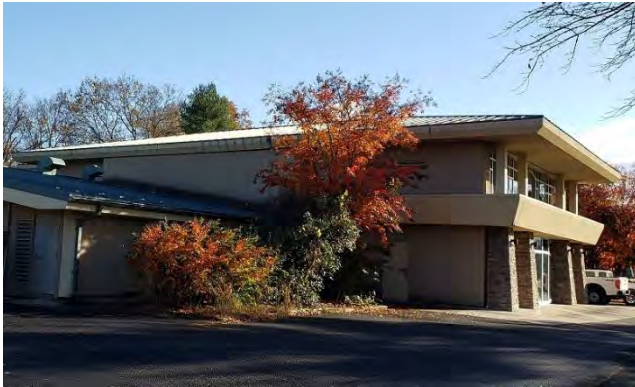
E-9: Roof 3 – West
