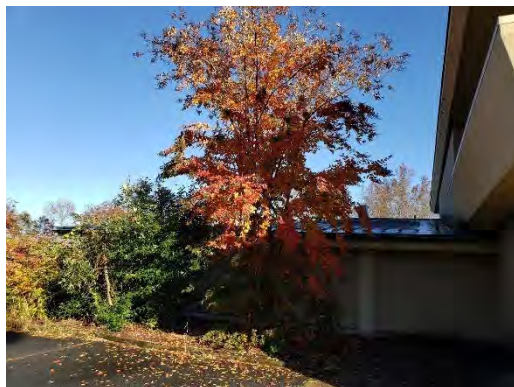
E-11: Roof 4 – East
