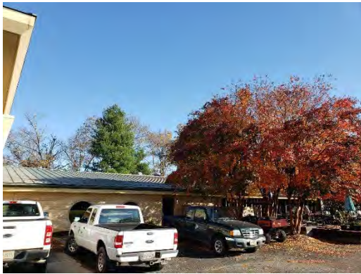
E-5: Roof 1 – West
