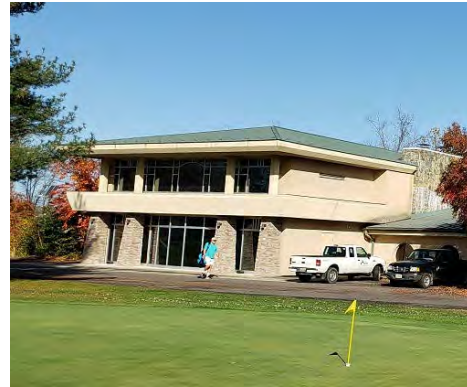
E-10: Roof 3 – South/East
