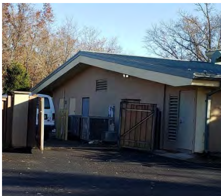
E-16: West Exterior Wall
