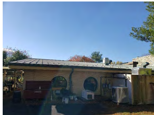
E-8: Roof 2 – East
