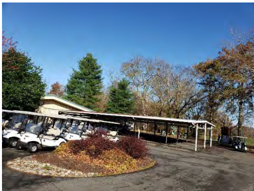
E-14: Roof 6 – Overall
