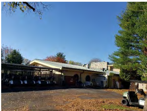
E-7: Roof 2 – Overall
